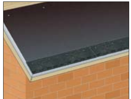
Install Leading Edge starter strips along the eave before installing the first course of shingles.
